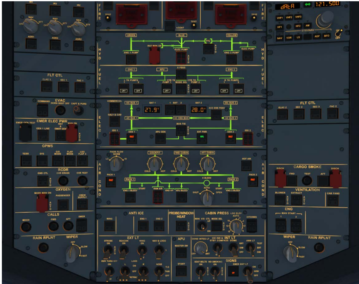
Picture 82: Overhead Panel before switching OFF both batteries
