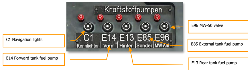
Figure 86: Circuit breakers of additional panel
